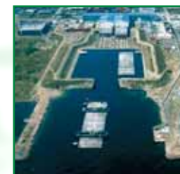
Figure 19. Example of Casting Basin (Öresun, Denmark)
