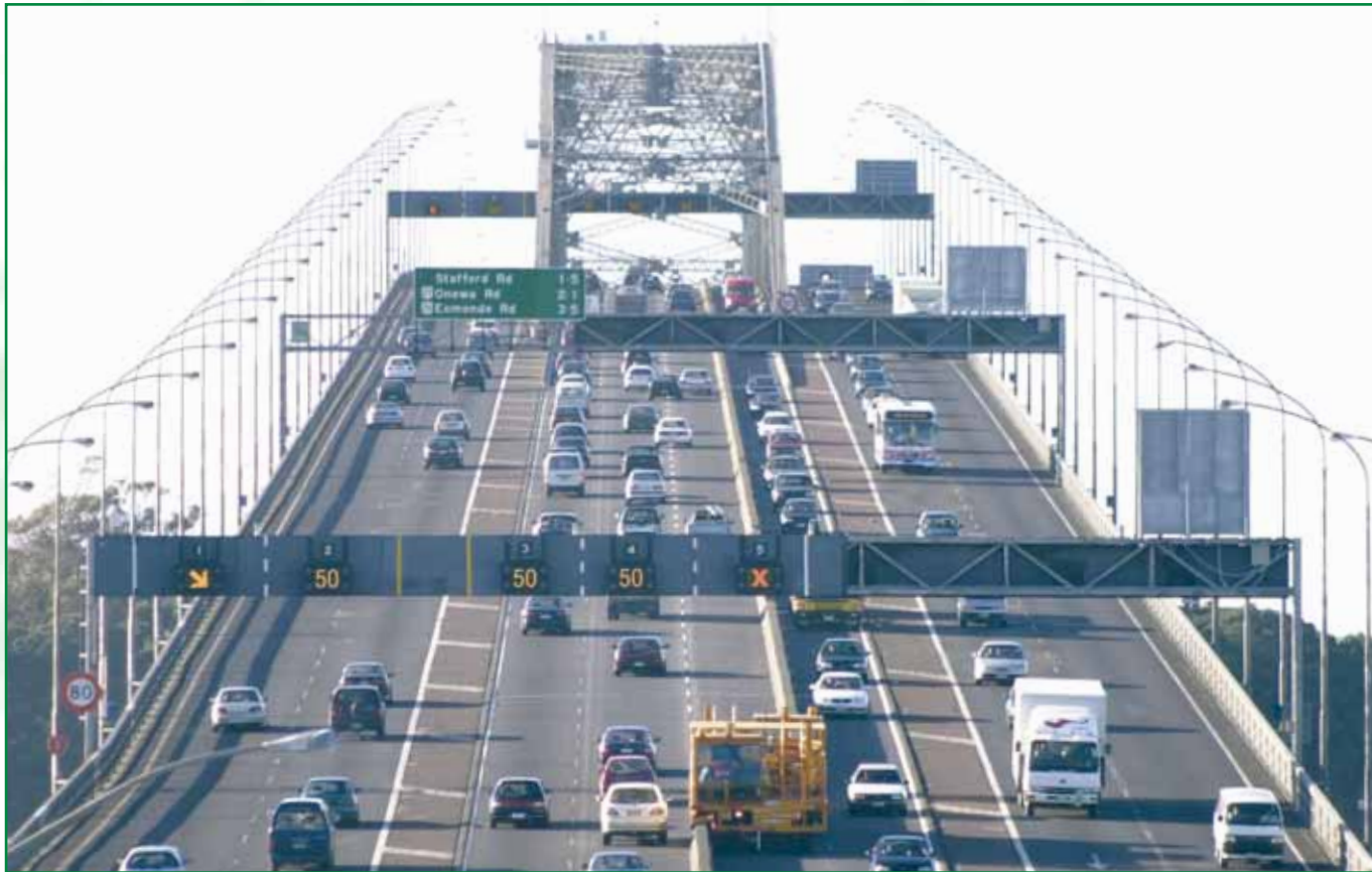
Figure 17. Auckland Harbour Bridge
