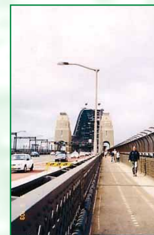
Figure 16. Footpath/Cycle Lane on Sydney Harbour Bridge
